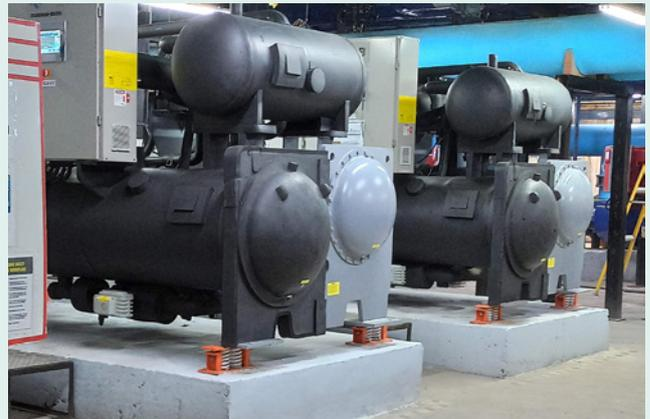
Chiller plant rooms with interconnecting chilled water header pipes
